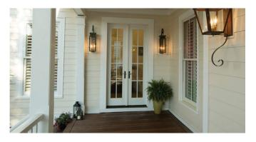
excels. The boards are made in 16-foot lengths as opposed to James Hardie's 12-foot board lengths. The end result is 33% fewer seams on your home when the product is installed. Fewer seams adds durability as well as beauty.
