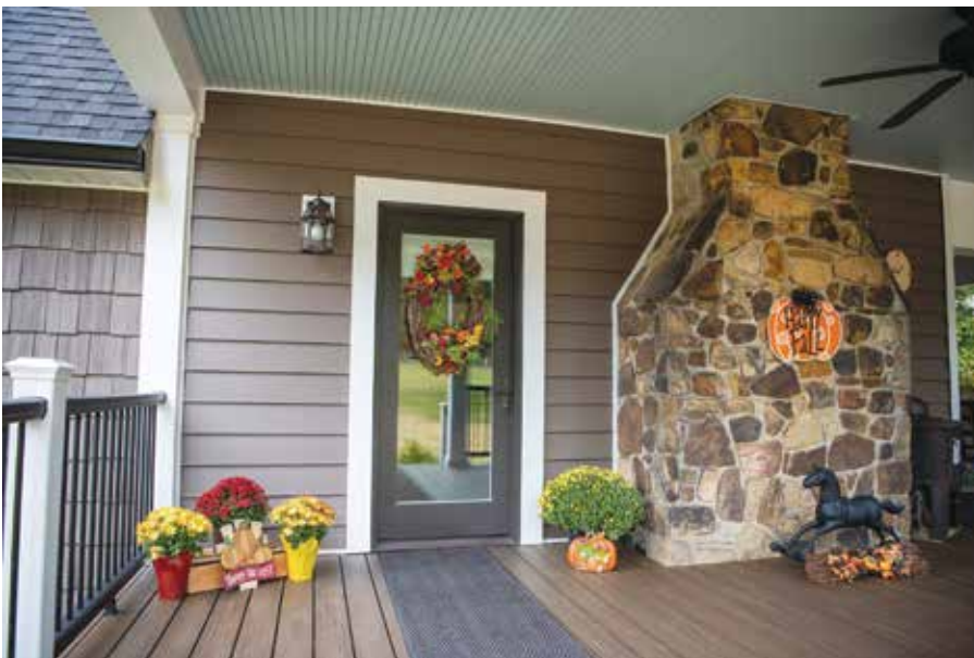
ABOVE: The new exterior elements include a vinyl ceiling in a traditional soft blue, Hardy Board siding and a synthetic Cedar shake. The decking is TREX and the original stone fireplace anchors the space.
